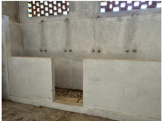
Changing room have been revamped and new showers installed.
