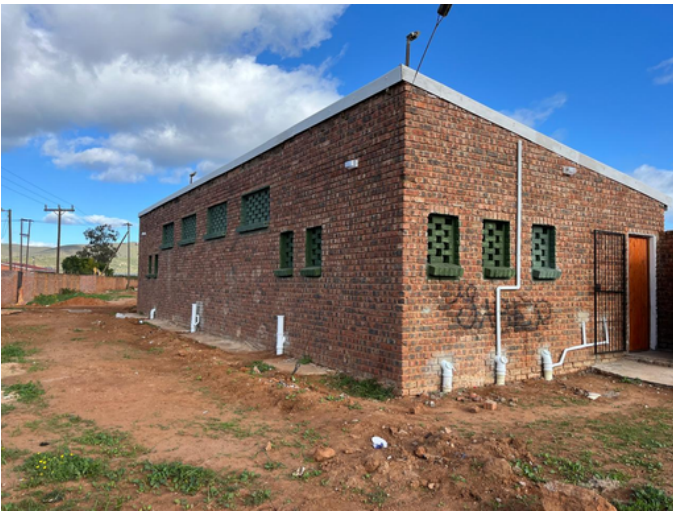
Windows have been restored.
