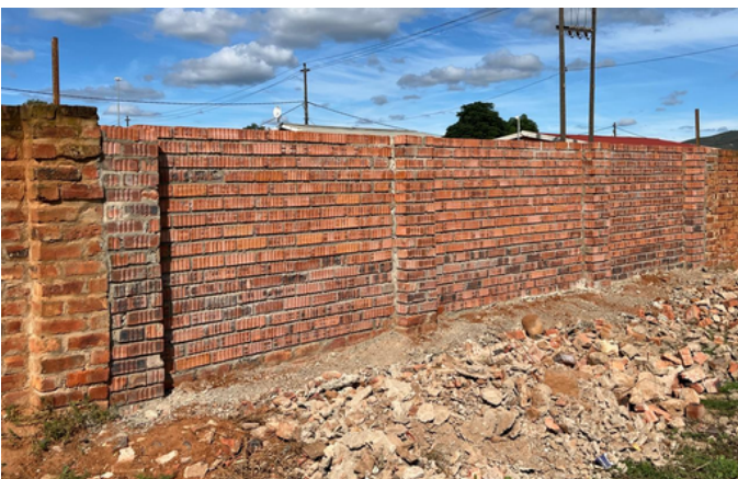
Boundary walls have been restored.
